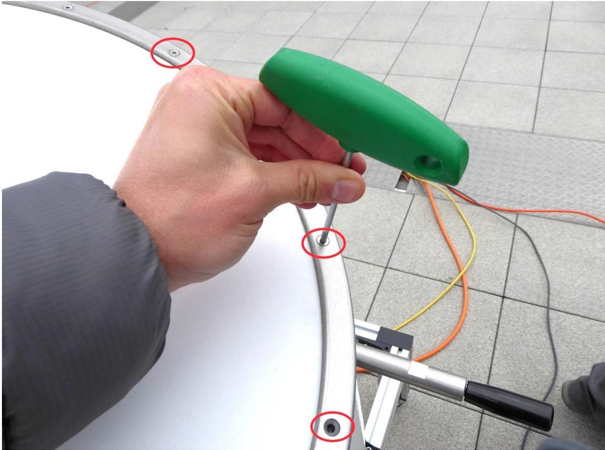
Remove the metal ring and the old radome material.
