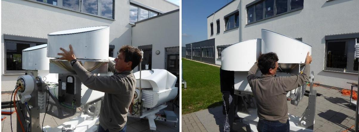
Install the blower air guides and tighten the flange screws:
